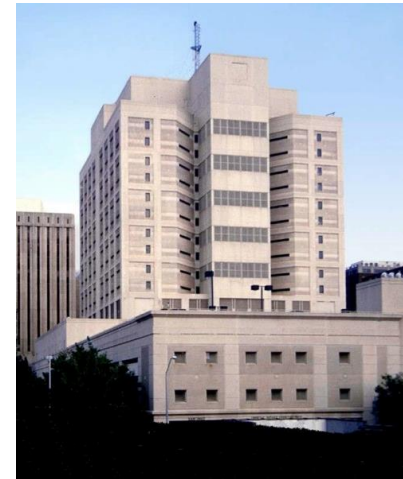
Public Safety Center
